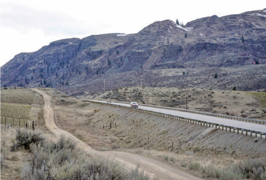
Fencing along highway 97 helps protect and guide animals.
