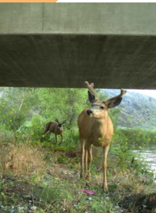
▲ Bucks using the Janis Bridge underpass. CWMP
