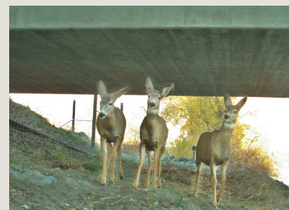
Three mule deer does crossing safely under Janis Bridge
