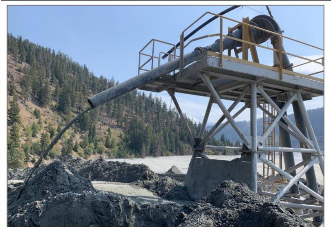
Photo 16: Cyclone discharging underflow (cyclone sand) on downstream face of West Dam
