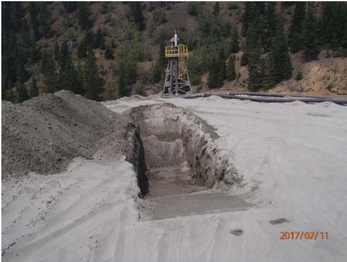
Photo II-2 Test pit excavation on the West Dam crest (ND17-WD-01)
