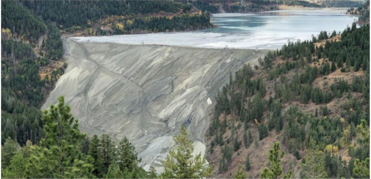
Figure 3a. At the end of 2022, the crest of the East Dam will be 973 meters above sea level, corresponding to an approximate height of 172.5 meters. The permitted crest elevation of 997 meters above sea level (corresponding to an approximate height of 196.5 meters) will be achieved in 2027. Photo from Klohn Crippen Berger (2021).
