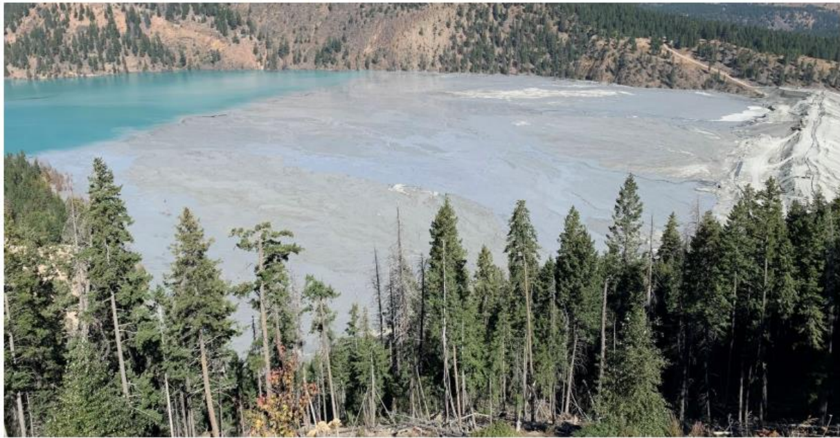
Figure 17b. The overflow from the cyclones (see Fig. 16) consisting of finer tailings and water is discharged from the crest of the East Dam toward the interior of the tailings management facility. The coarser fraction of the overflow settles closer to the dam crest to form a tailings beach (middle to right-hand side of photo; compare with Figs. 2 and 11). The finest fraction of the overflow (slimes) is carried to the interior of the tailings management facility (left-hand side of photo; compare with Figs. 2 and 11). Photo from Tetra Tech (2022).
